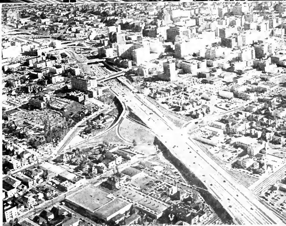
Looking northeasterly from above Las Angeles showing completed portion of the Harbor Freeway extending from foreground right to center left. Downtown business district and Civic Center shown center and right. The grade separation bridge, foreground right, carries Olympic Blvd. under the Harbor Freeway. Next above Olympic Blvd. is Ninth St. that carries one-way traffic eastbound, and above it is Eighth St. which carries one-way traffic westbound.
